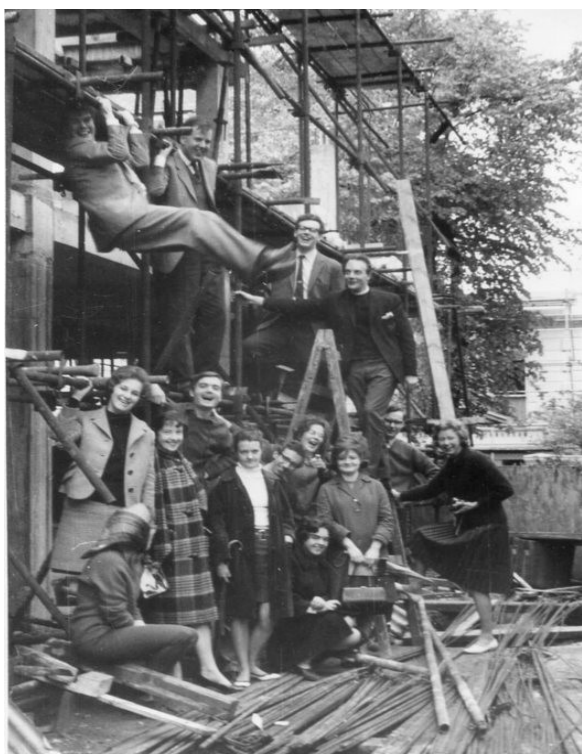
The Under 30's group hanging onto the scaffolding for the new church hall - Photo from Sheila Gibbs
