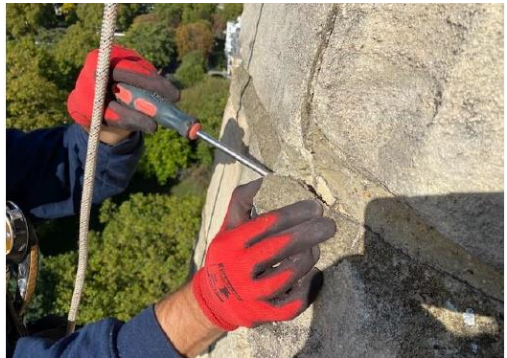
Work on Spire: photo by Braileys Ltd 1
